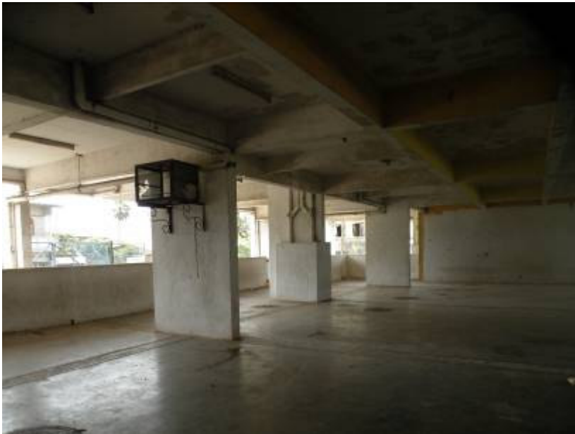
Figure 2: Sahasthipura Community Centre at the present
